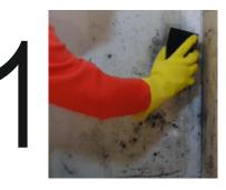
Apply "FK-12 Gel" dampness cleaner generously to the affected area with a brush, rub with the scrub pad and leave to act for 5 minutes. Then remove inconsistent parts, and rinse with the sponge and clean water. Allow to dry completely. If necessary, repeat the operation until the surface no longer shows any damage.
