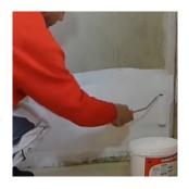
After the primer has dried, apply 2 to 3 coats of DISPERLITH Industry paint by brush or roller to provide a paint film with high resistance to moisture, mold, mildew, bacteria, biofilm and viruses.
