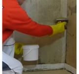
After the previous cleaning and sanitation process, apply undiluted and on the dry surface, the penetrating primer "Disperlith Primer", which will increase the resistance to moisture, mold and microorganisms from the inside of the base, while providing an adequate adhesion of the subsequent paint.
